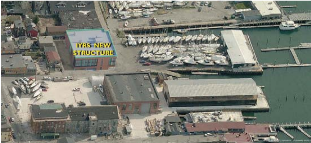
FIGURE 3: AERIAL VIEW OF THE INTERNATIONAL YACHT RESTORATION SCHOOL (IYRS) OF TECHNOLOGY & TRADES NEWPORT, RI CAMPUS. THE CAMPUS IS SITED WITHIN A LIVELY WORKING WATERFRONT DOWNTOWN BUSINESS DISTRICT AND FRONTS HISTORIC THAMES STREET. THE NEW STRUCTURE FOR MARINE SYSTEMS AND COMPOSITES PROGRAMS IS SITED NEXT TO THE EXISTING IYRS FACILITIES ON SPRING WHARF. THE PROGRAM FOR THE BUILDING INCLUDES CLASSROOMS AND TRADE TEACHING AREAS FOR MARINE SYSTEMS, COMPOSITES AND DIGITAL FABRICATIONS ON TWO UPPER FLOORS ABOVE OPEN PARKING, WHICH IS AT THE BOATYARD LEVEL WITHIN THE FEMA ZONE VE SPECIAL FLOOD HAZARD AREA (AREAS OF FLOODING WITH ADDITIONAL HAZARDS DUE TO STORM-INDUCED VELOCITY WAVE ACTION). PHOTO CREDIT: WILSON ARCHITECTS.
