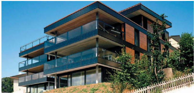
FIGURE 5: NET POSITIVE ENERGY PROJECT, "HOFBERG 6/7" IN WIL, CANTON OF ST. GALLEN, SWITZERLAND. RECIPIENT OF THE 2012 LORD NORMAN FOSTER SOLAR AWARD. BUILDING IS MINERGIE-P® CERTIFIED (SG-074-P) AND PRODUCES ROUGHLY 180 PERCENT OF ITS TOTAL ENERGY DEMAND. ARCHITECTURE BY FENT SOLARE ARCHITEKTUR. PHOTO CREDIT: LUCIDO SOLAR AG.
