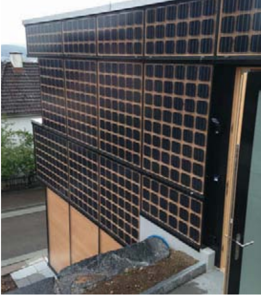
FIGURE 7: NET POSITIVE ENERGY PROJECT (121 PERCENT), HOFBERG 8 (2016) IN WIL, CANTON OF ST. GALLEN, SWITZERLAND WITH SAF® E3. MINERGIE-P CERTIFIED (SG-125-P). ARCHITECTURE BY FENT SOLARE ARCHITEKTUR. PHOTO CREDIT: LUCIDO SOLAR AG.
